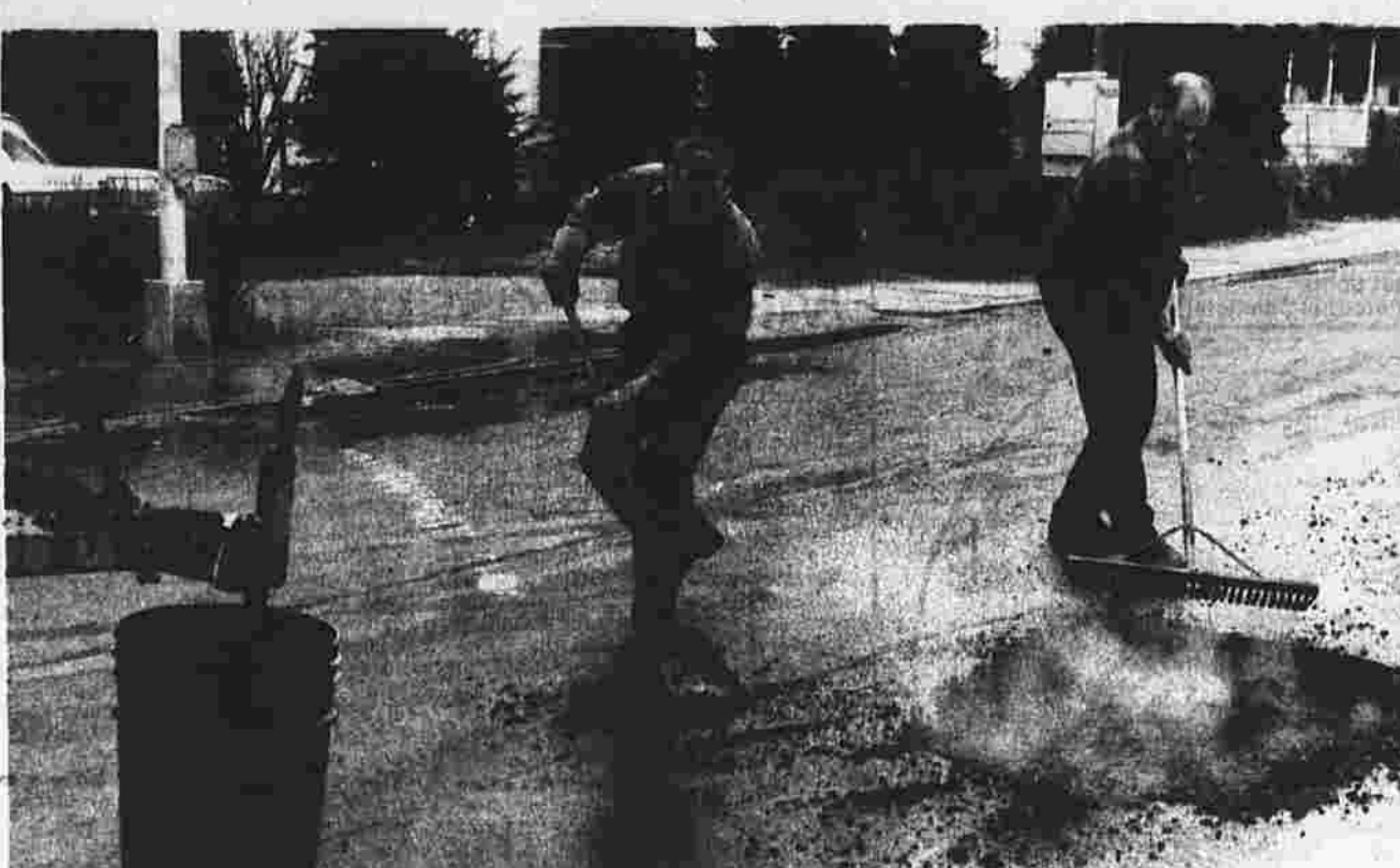
After the rain George Hewitt (left) and Earl Keney fill in a pothole on Spruce Street. They work for the town highway department, which has its work cut out for it these days on the town's pock-marked streets.
